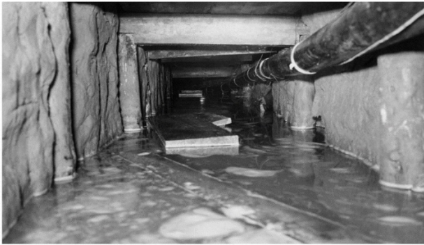
The old, flooded tunnel
